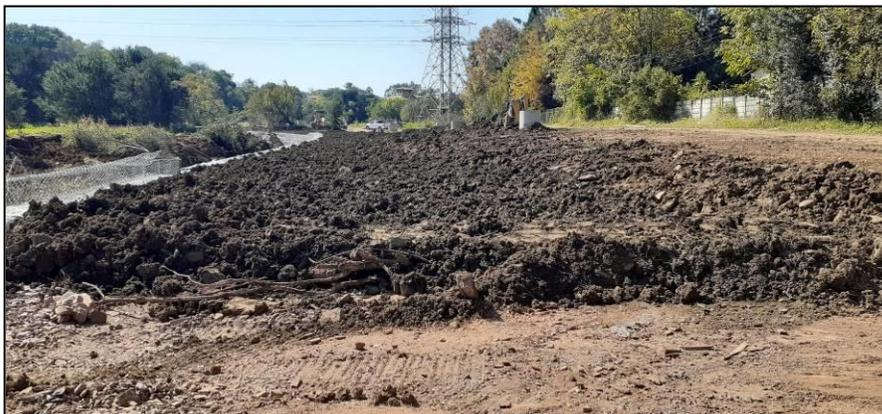
More soil was used to cover the shotcrete-protected pipeline and fill in up to the gabions along the new river bank. There are questions as to the necessity of moving the river bed quite so far.
