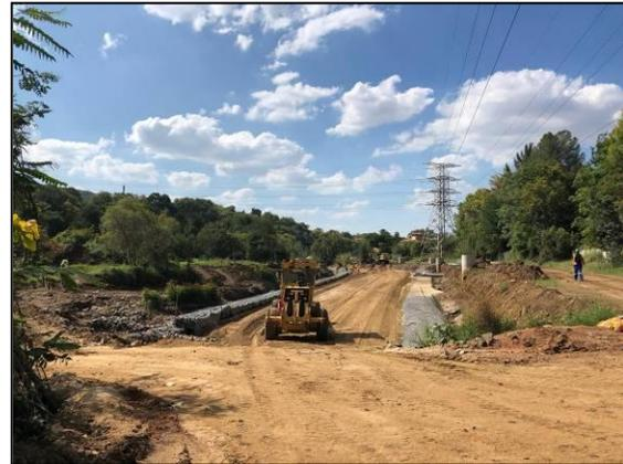
*Above left:* the pipeline was supported by sandbags and the river was moved about five metres to the west. Here rock was being dumped in former river bed. *Right:* the sandbagged pipeline on right of the vehicle is now covered by shotcrete and soil is being compacted over the dumped rock. Gabions left of the vehicle mark the new river bank.
