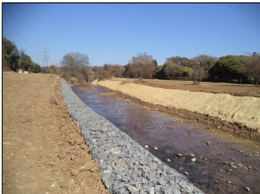
In August we were able to visit the site and found that the river now looked like a canal. Despite recommendations to have banks sloped at 1:3 or 1:4, the sides were made very steep and covered by 200 metres of gabions on the pipeline side and Geomesh (not planted with any vegetation) on the other. Thirty metres of gabions were installed on both sides at the downstream end where the pipeline crosses under the river.
